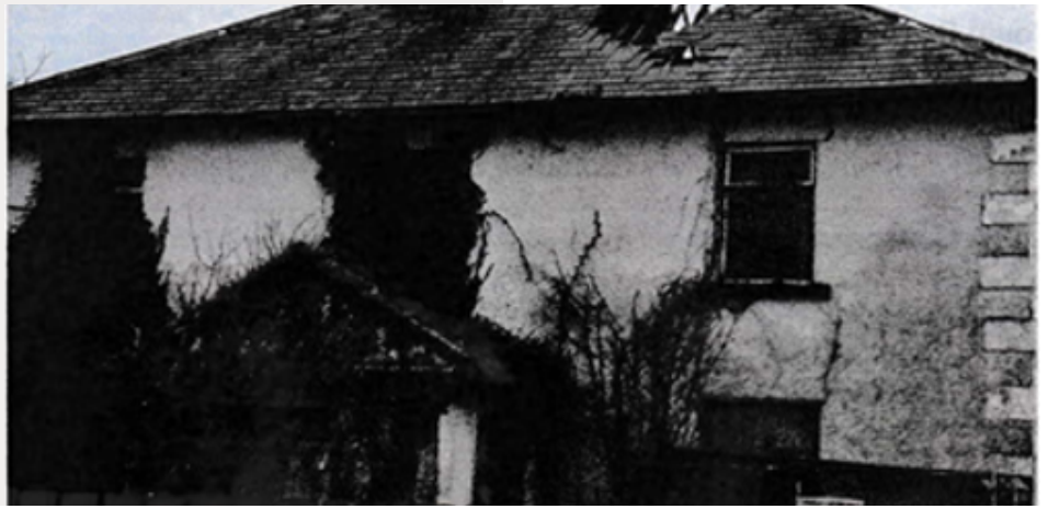
Pictured: The Killygordon Youth Club before refurbishment
